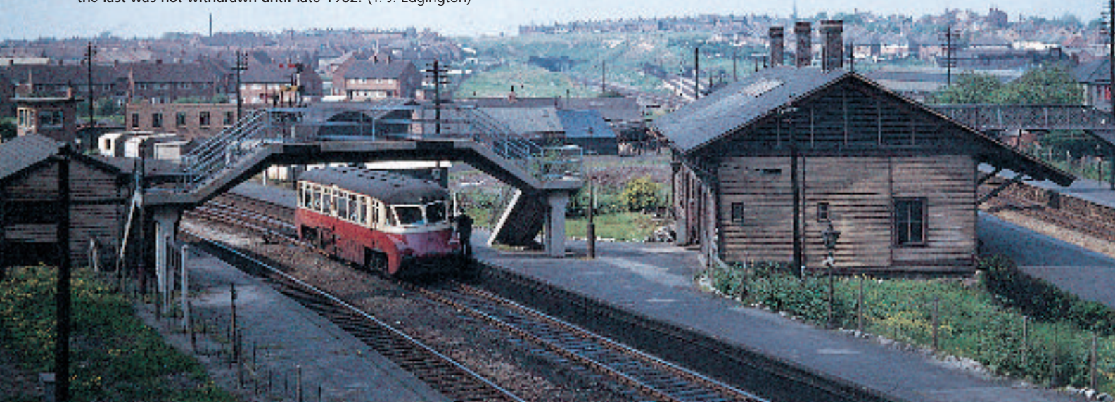
BELOW: The logical next step was to produce a twin-car unit and the Great Western introduced two such pairs in 1941/2, Nos.35/36 and 37/38. These featured a buffet counter and were intended to replace single cars on the Birmingham–Cardiff run but in fact were so successful in attracting passengers that conventional steam trains of greater capacity had to take over the service! They were capable of running with
